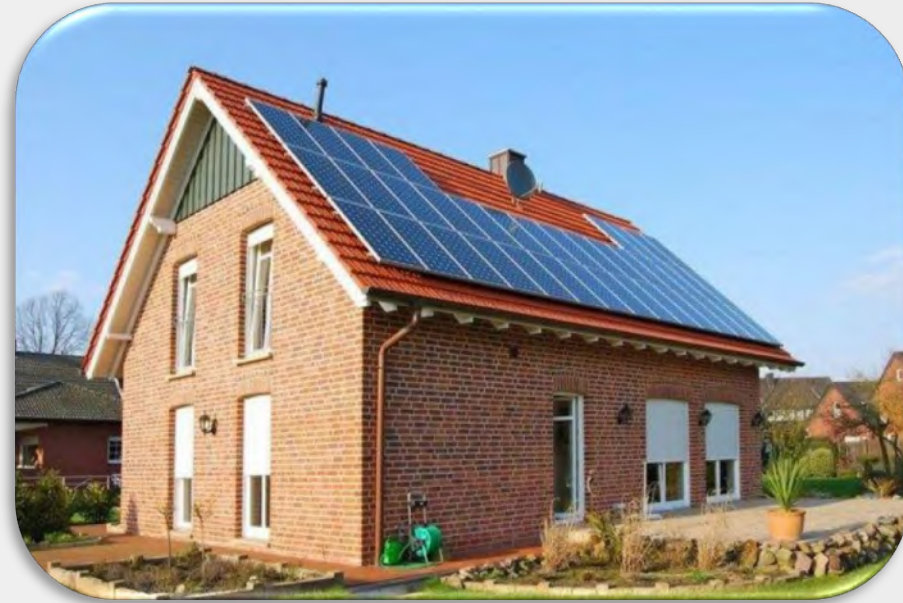
500kw Roof System Germany year 2014
