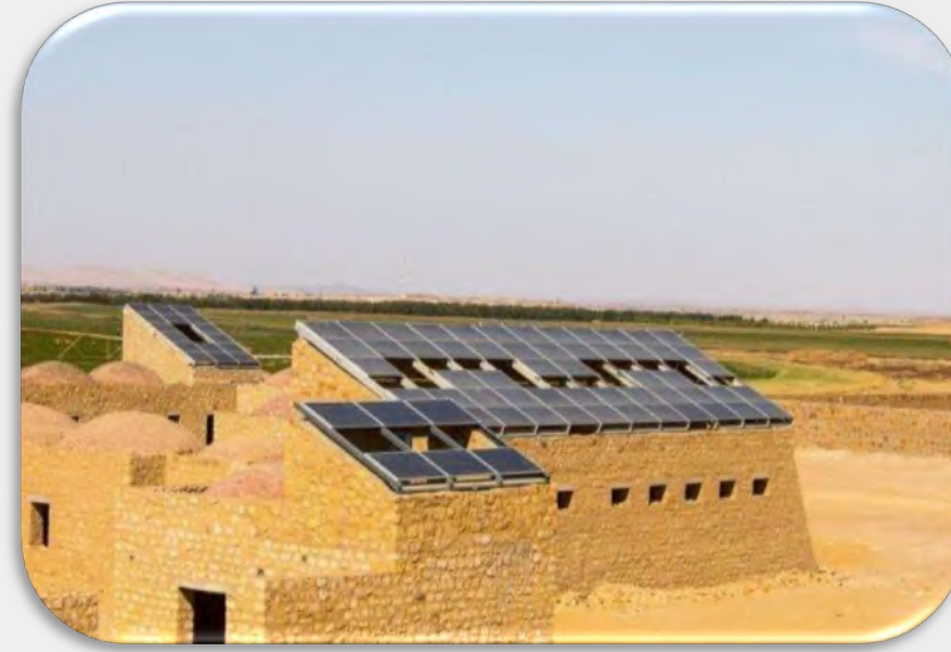
200kw Solar System Morocco year 2018
