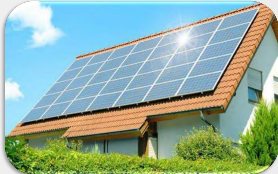
800kw Roof System Netherlands year 2014
