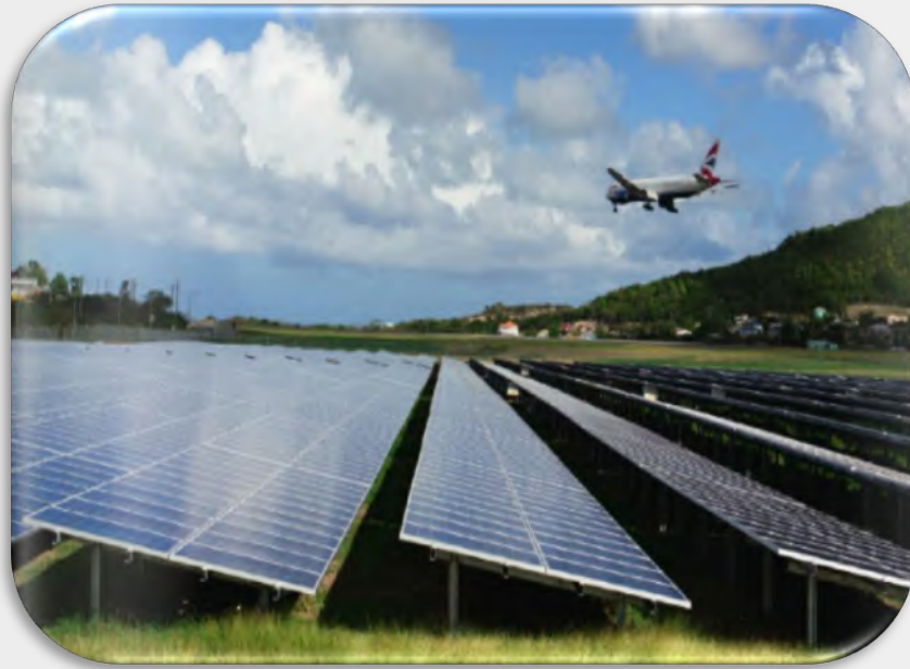
3MW Solar Power PV Station Antigua year 2016
