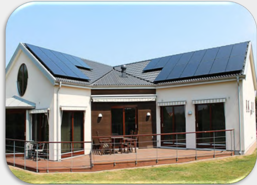
300KW Residential Roof Solar Power Sweden year 2016
