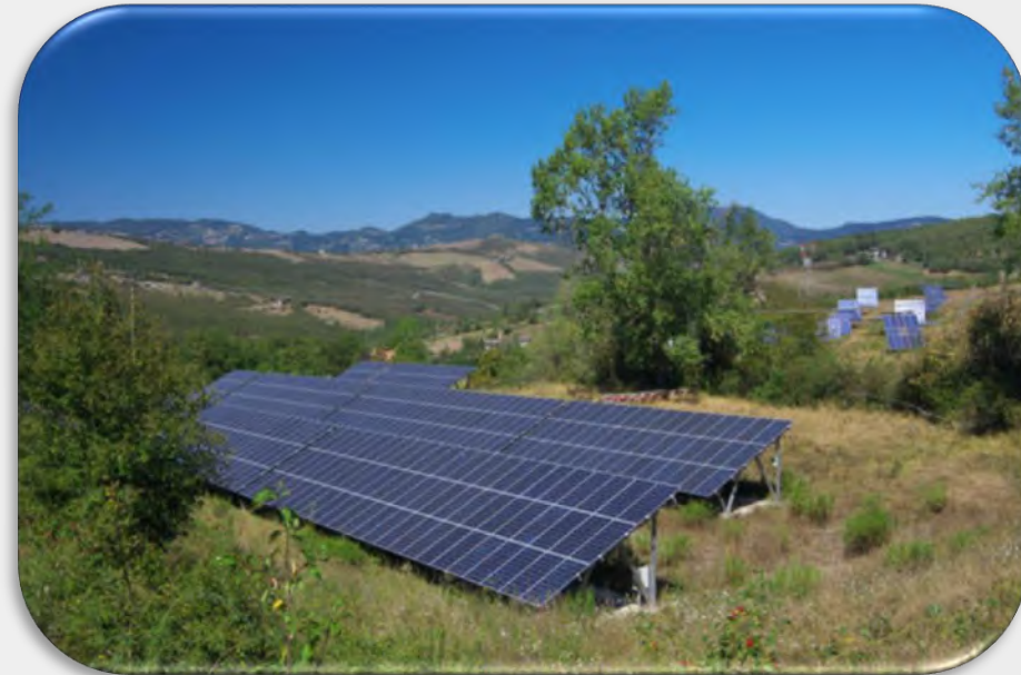
500kw Power Plant Italy year 2018
