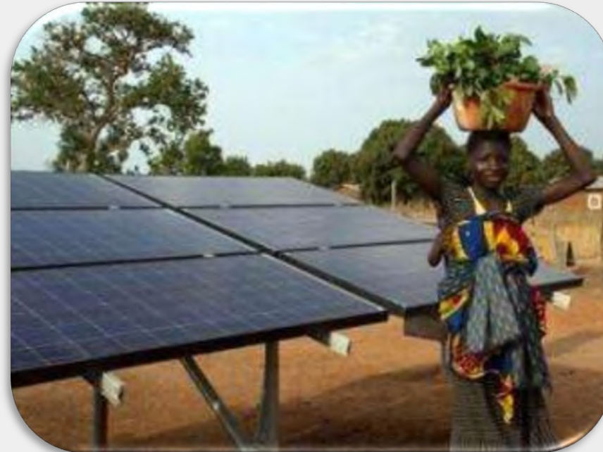
200kw Solar System Nigeria year 2018
