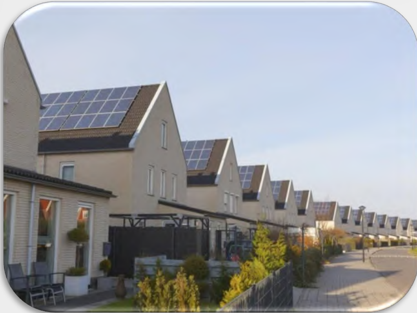
2MW Residential Roof System Germany year 2015
