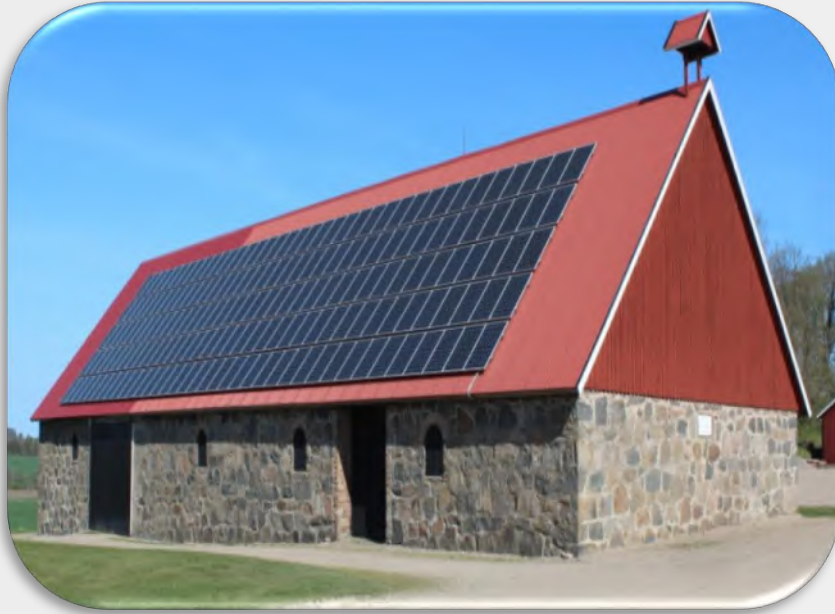
500KW Roof System Sweden year 2016
