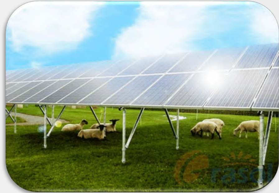
1MW Power Plant Switzerland year 2016
