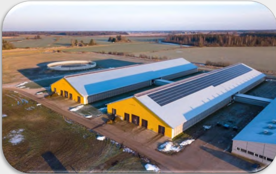
1.1MW Solar Power Plant Estonia year 2019
