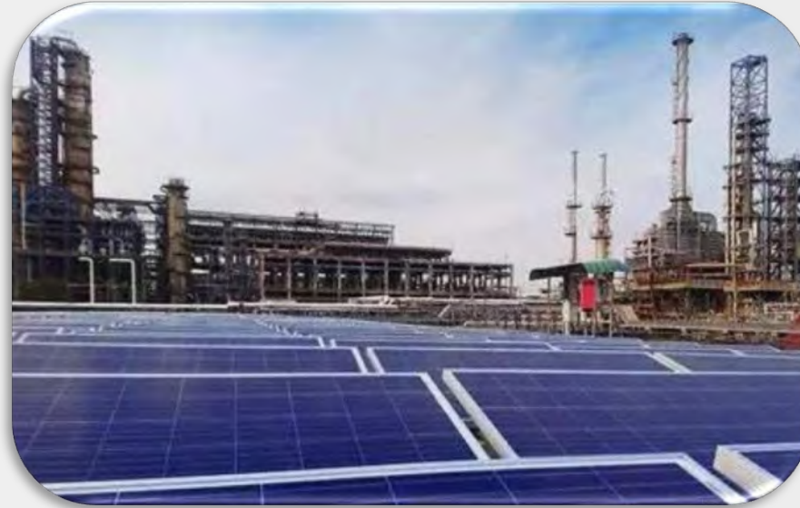
5MW Power Plant India year 2018
